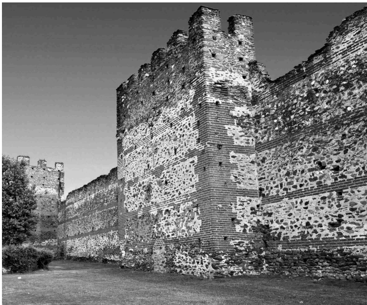
Figure 2.3 Section of the defensive walls of Thessalonica
